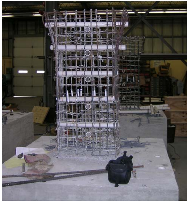
Figure 4.8: Column Reinforcement Cage
